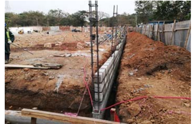
Camp Expansion – Boundary fence erection
