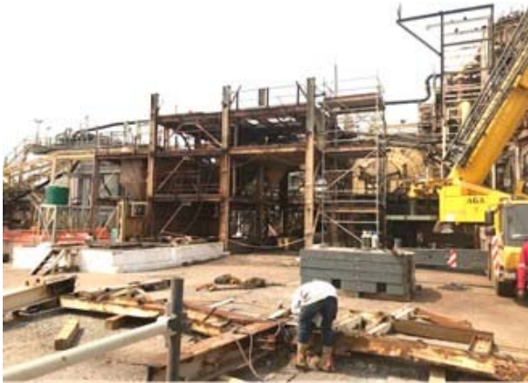
Gravity structure - Two levels removed
