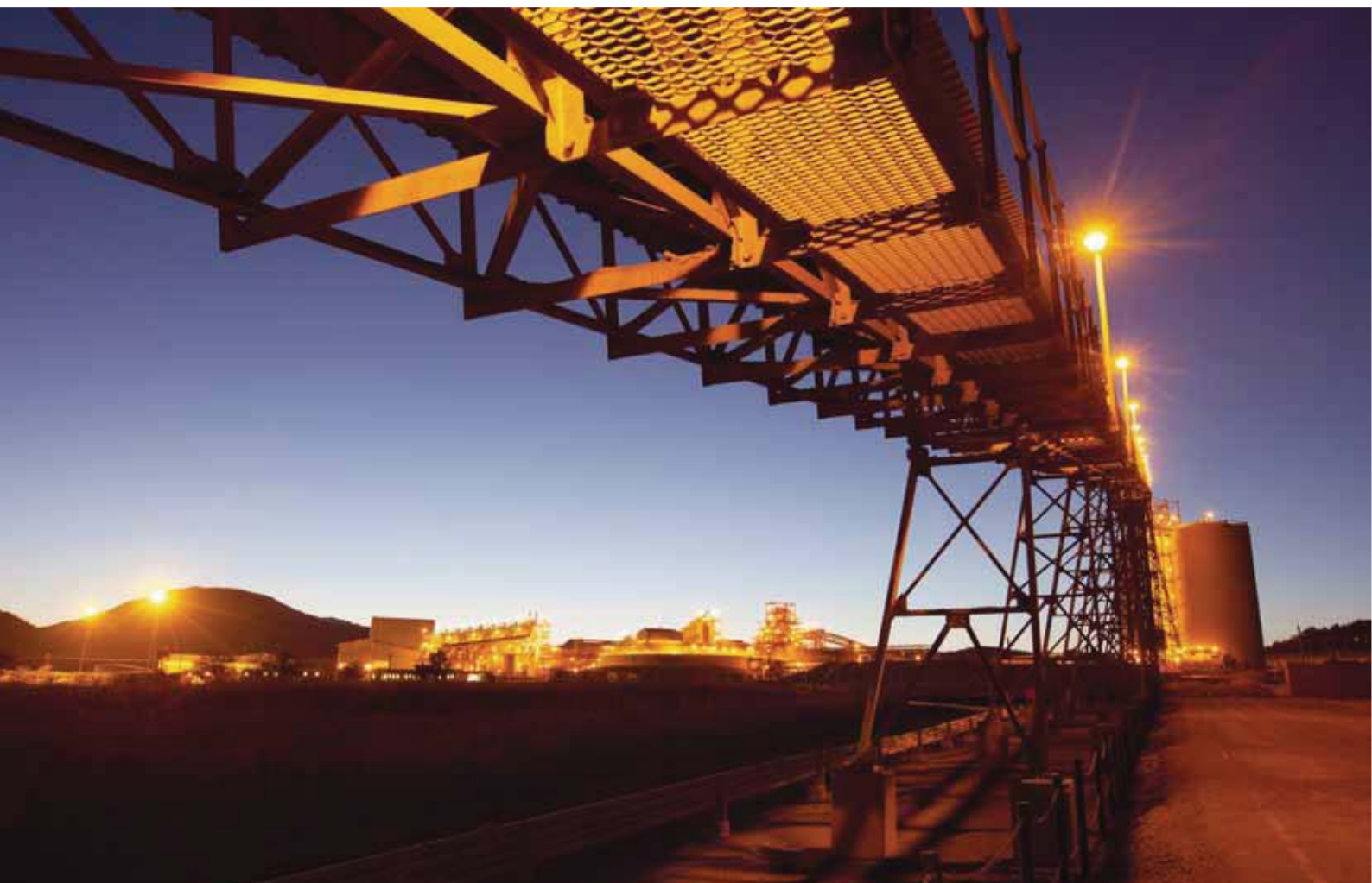
Two Rivers Platinum Mine overland conveyor belt towards primary and secondary crushers
