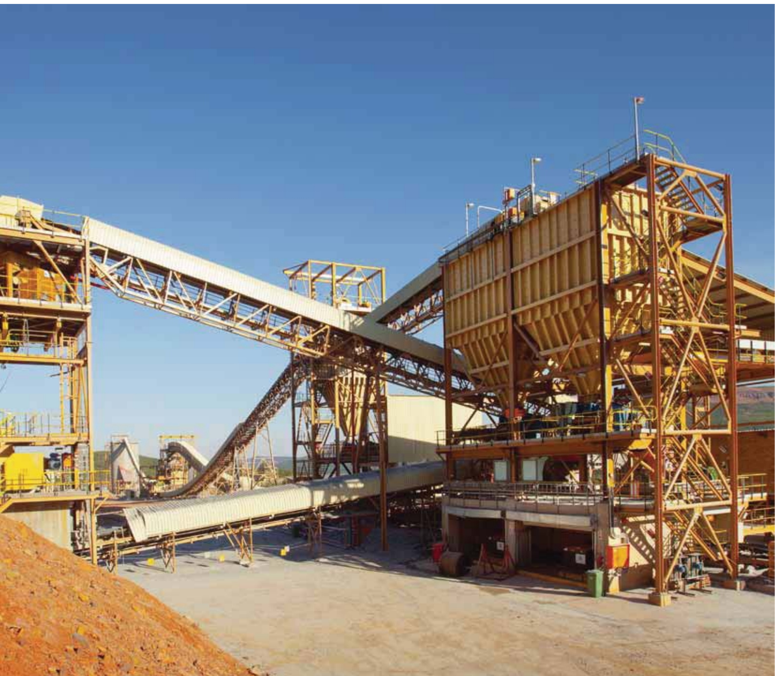
Nkomati Nickel Mine PCMZ concentrator plant Sandvik Crusher during construction
