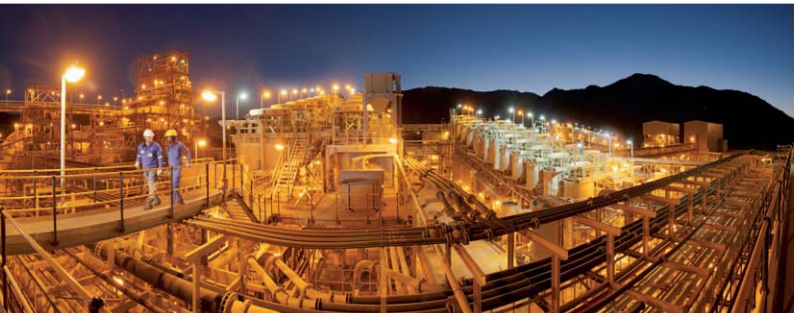
Two Rivers Platinum Mine flotation section
