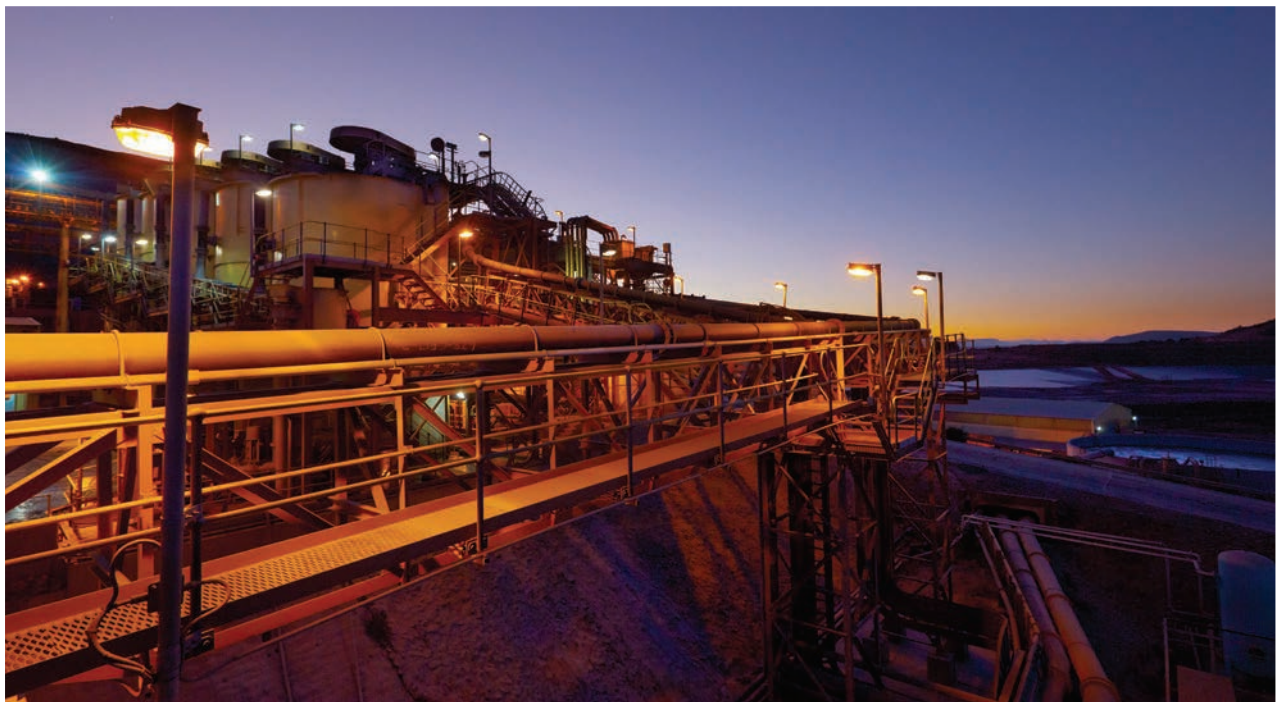
PCMZ plant, Nkomati Mine
