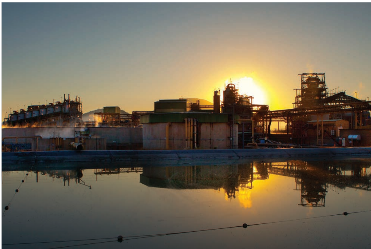
Two Rivers Platinum Mine silo's and conveyors
