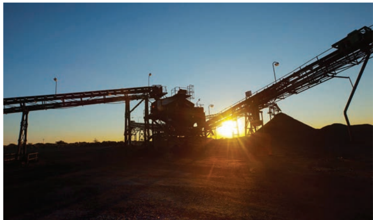
Gloria Manganese Mine plant
