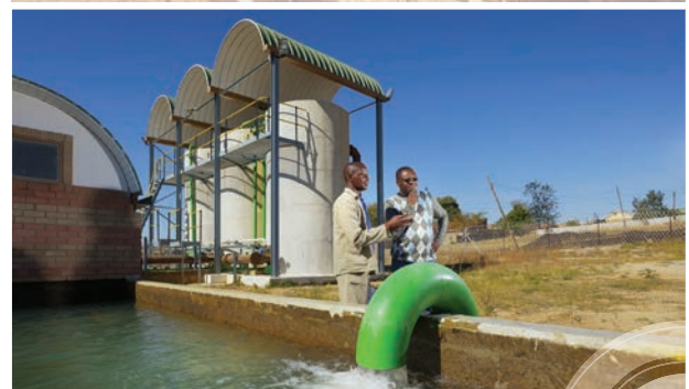
Badplaas water treatment plant upgrade, Nkomati Mine
