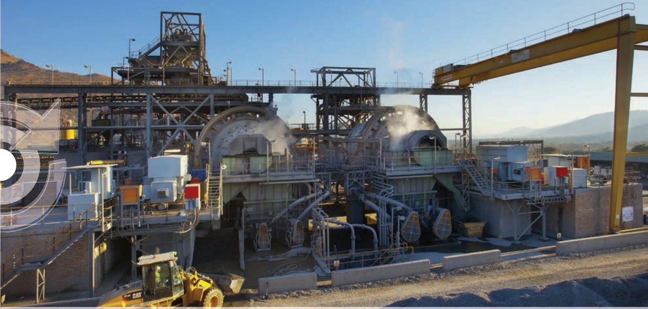
Concentrator plant at Two Rivers Platinum Mine
