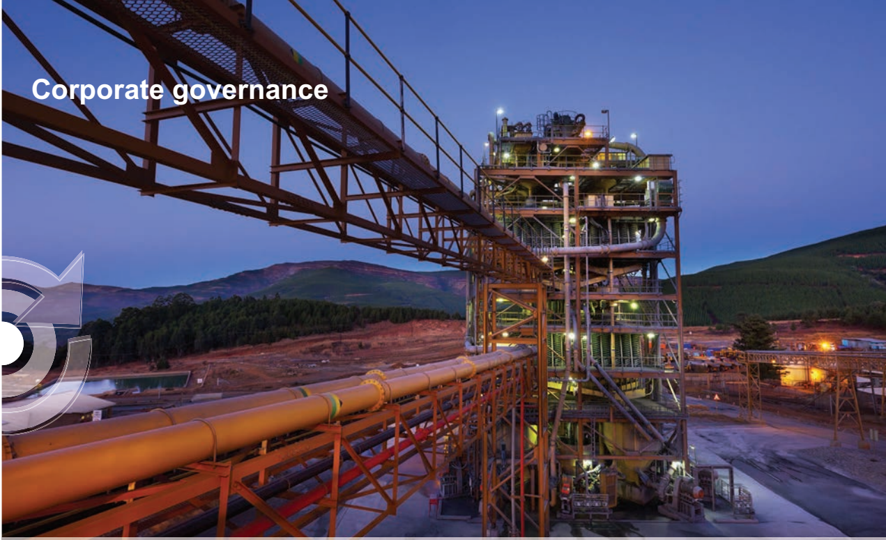
PCMZ Plant, Nkomati Mine
