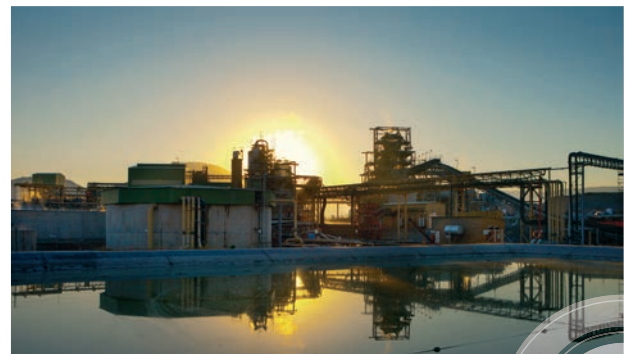
Two Rivers Platinum Mine
