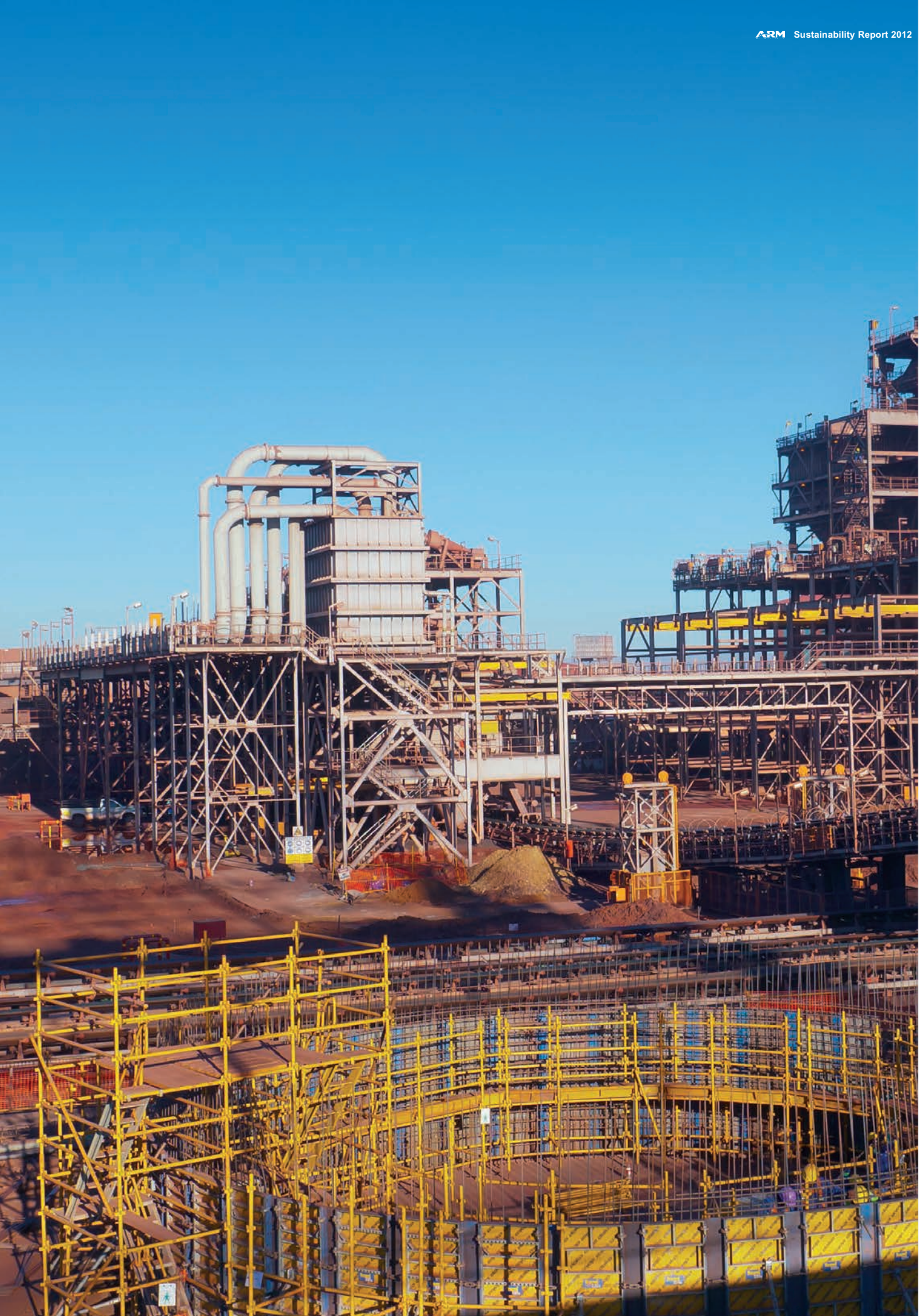
WHIMS plant under construction at Khumani Iron Ore Mine
