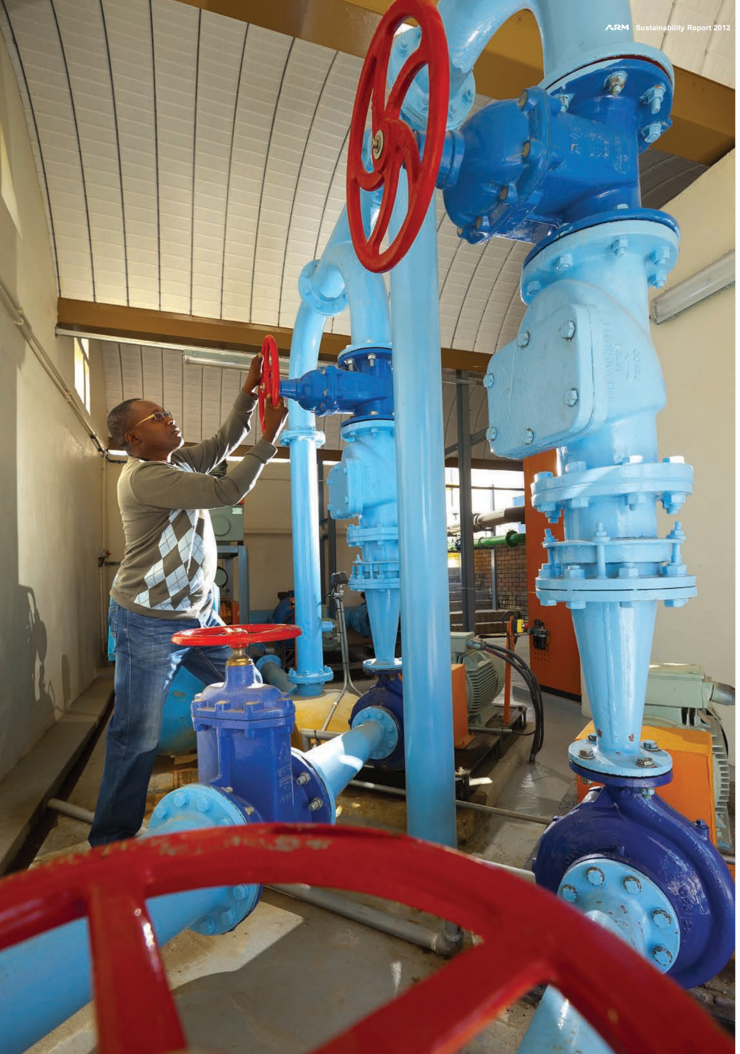
Badplaas water treatment plant upgrade, Nkomati Mine
