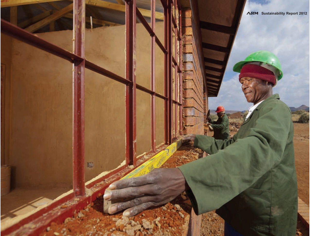
New building for home-based care, Black Rock Mine
