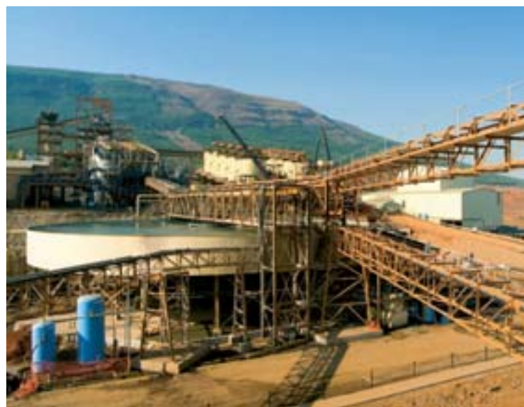
Tailings thickener Nkomati Nickel Mine
