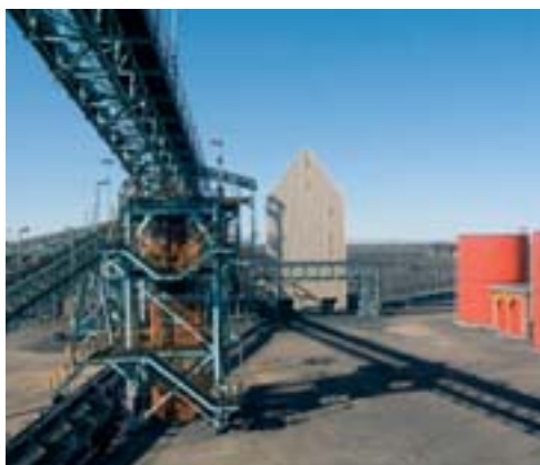
Khumani Iron Ore Mine sampling tower
