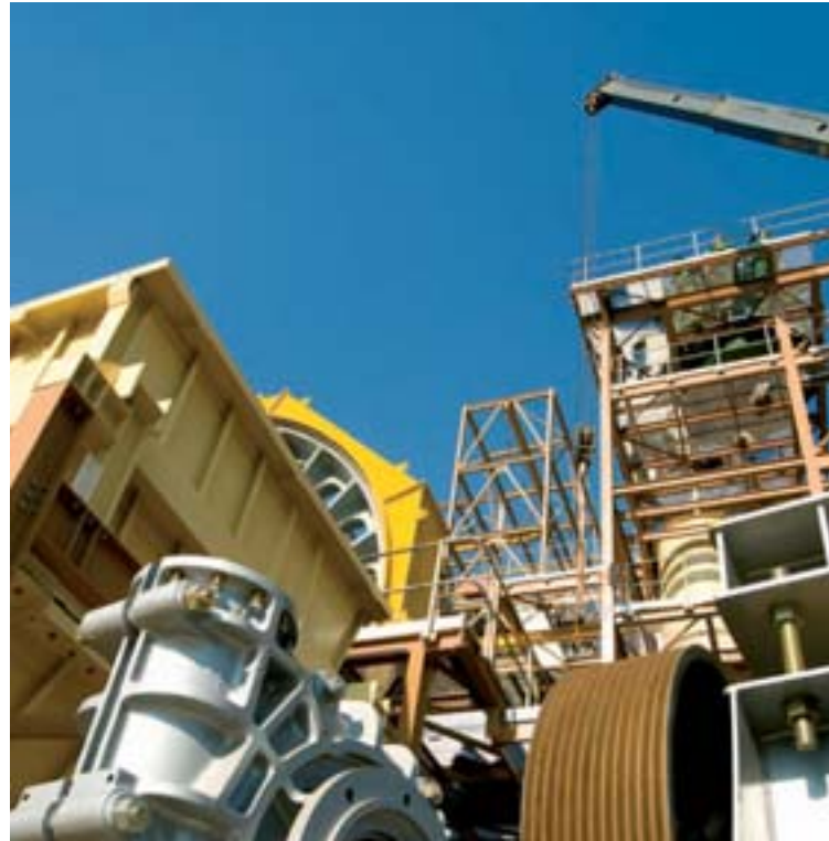
Nkomati PCMZ plant construction
