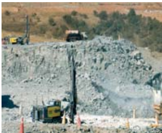
Nkomati open-pit blast hole drilling
