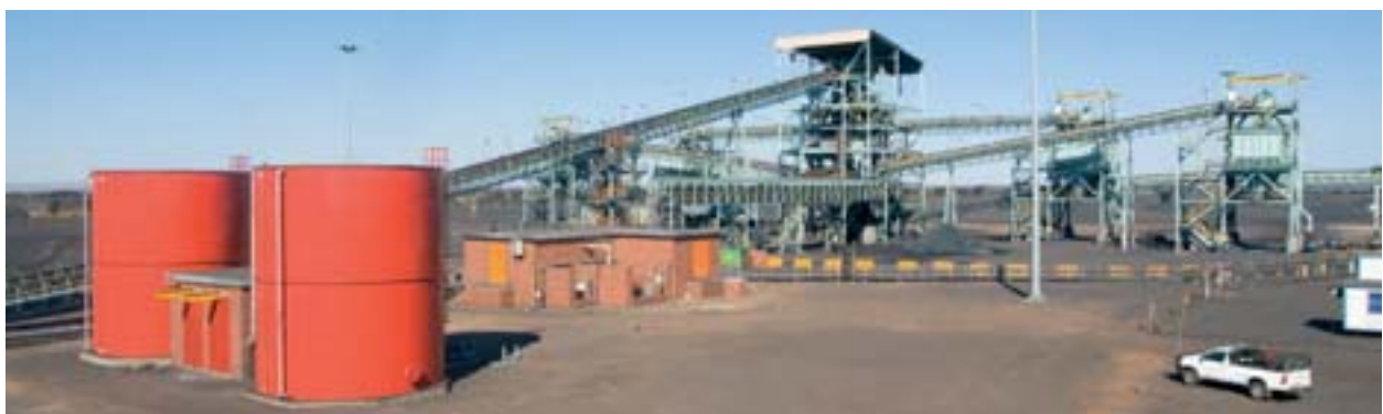
New Nchwaning processing plant
