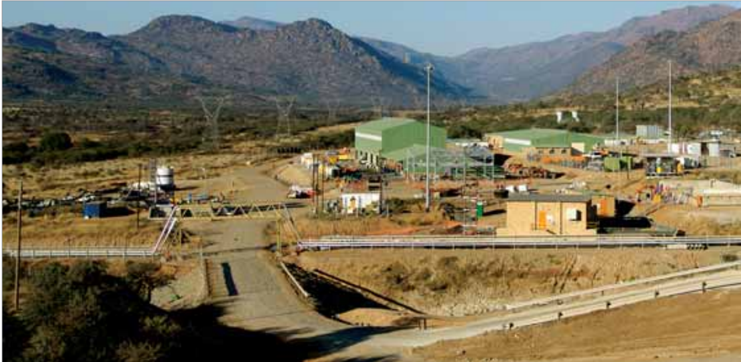
Two Rivers Platinum Mine
