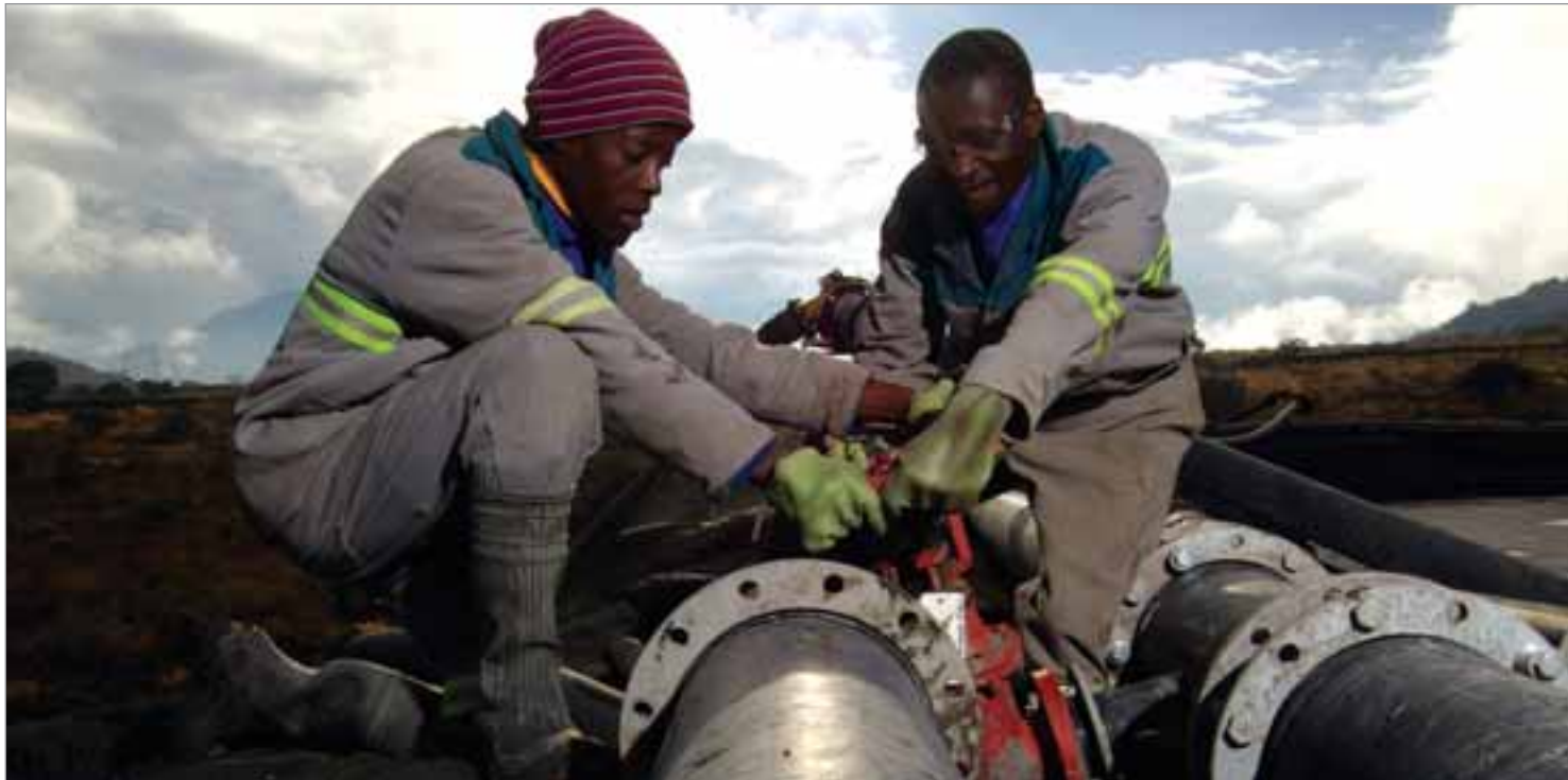
Two Rivers Platinum Mine
