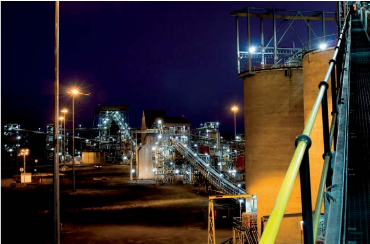
The new manganese ore crushing and screening plant at Nchwaning
