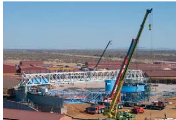
Construction of new thickener at Khumani
