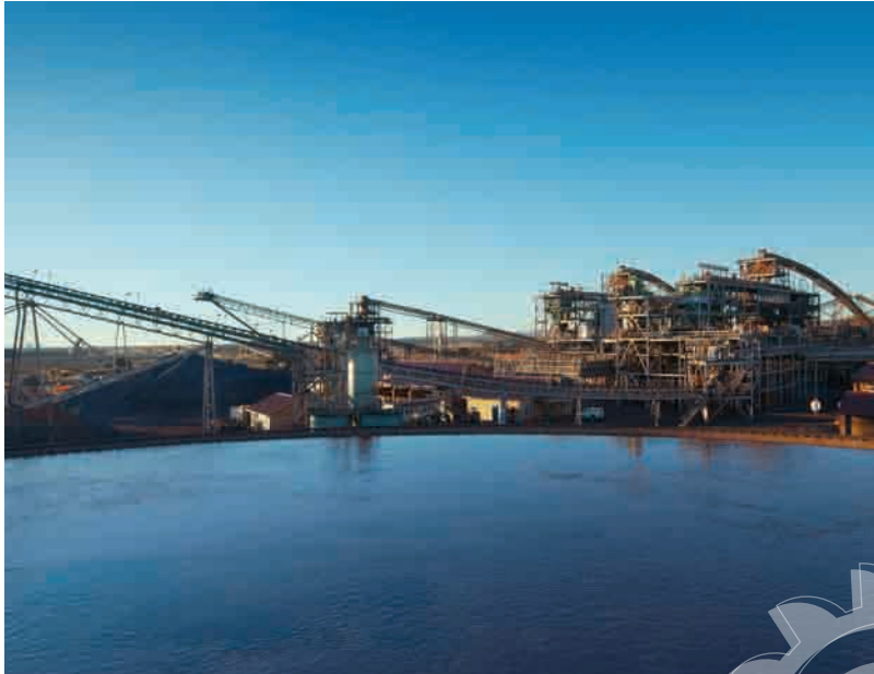
Parsons plant, Khumani Iron Ore Mine
