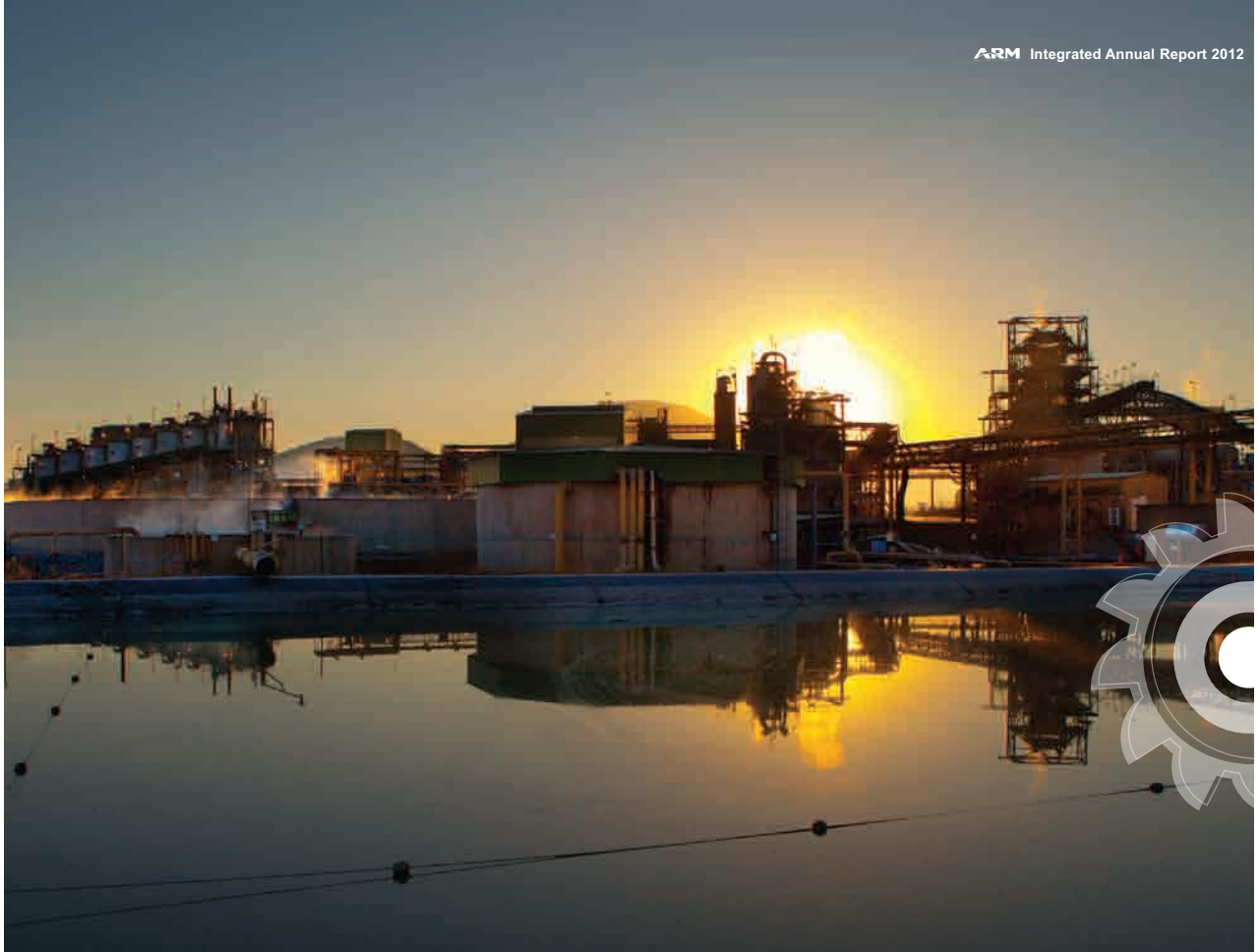
Two Rivers Platinum Mine silos and conveyors
