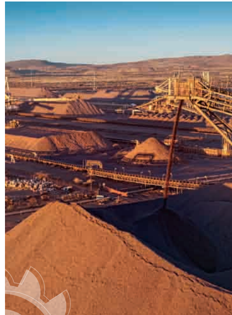
Parsons plant, Khumani Iron Ore Mine
