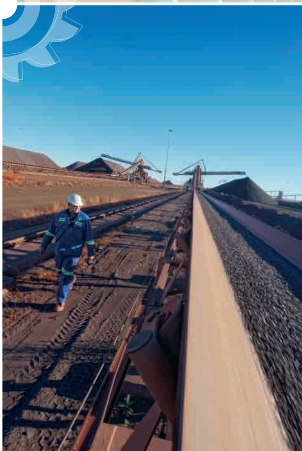
New load out station at Khumani Iron Ore Mine
