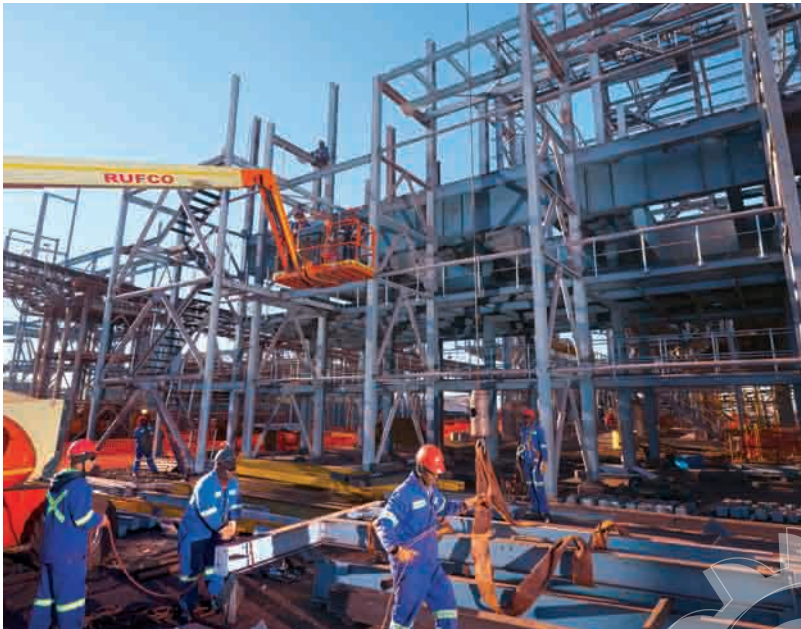
New WHIMS plant under construction at Khumani Iron Ore Mine
