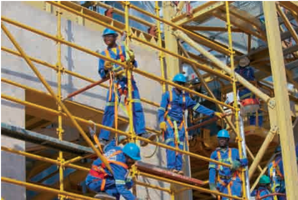
Construction of the concentrator plant at Lubambe Copper Mine
