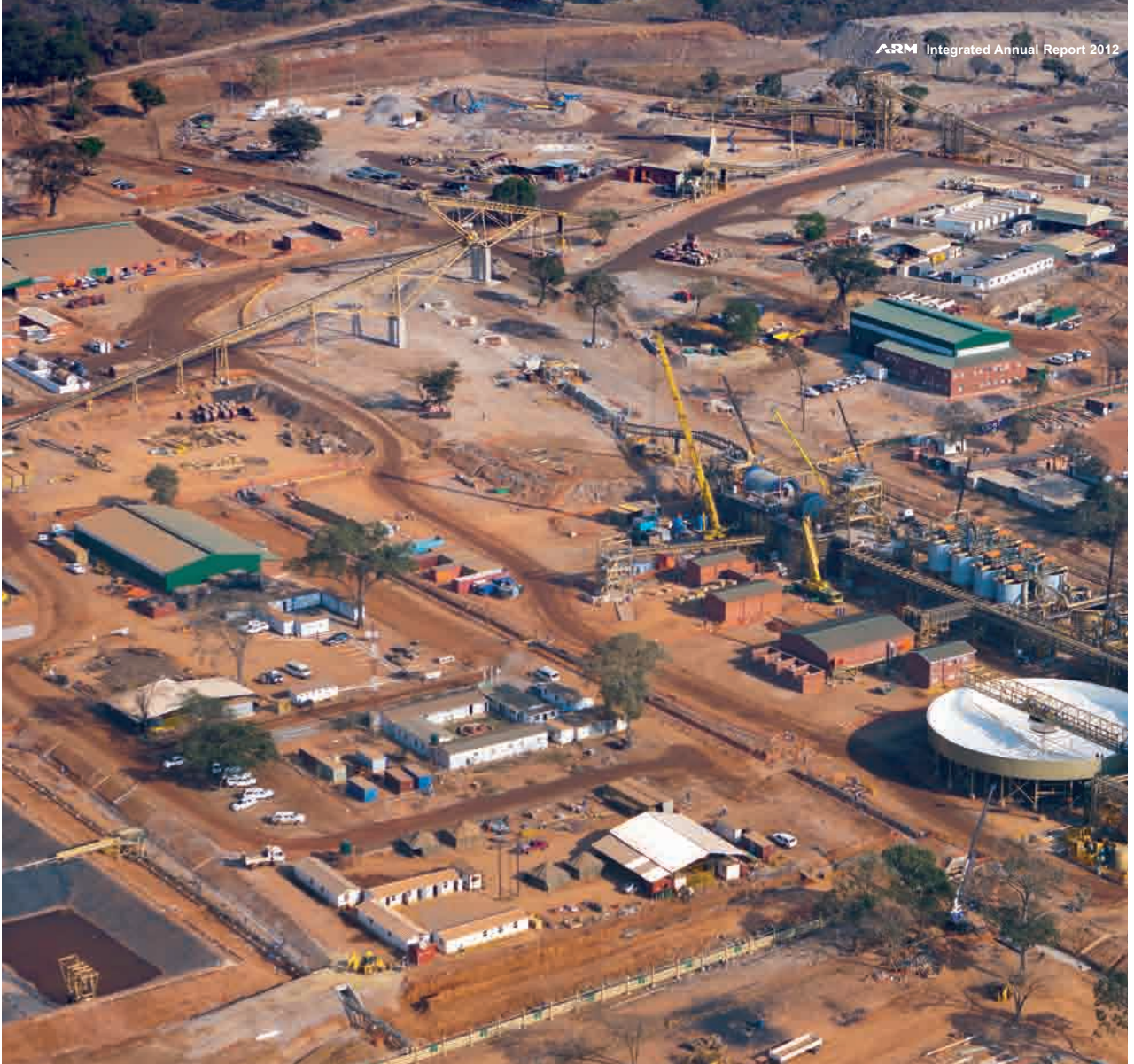
Aerial view of Lubambe Copper Mine and concentrator plant
