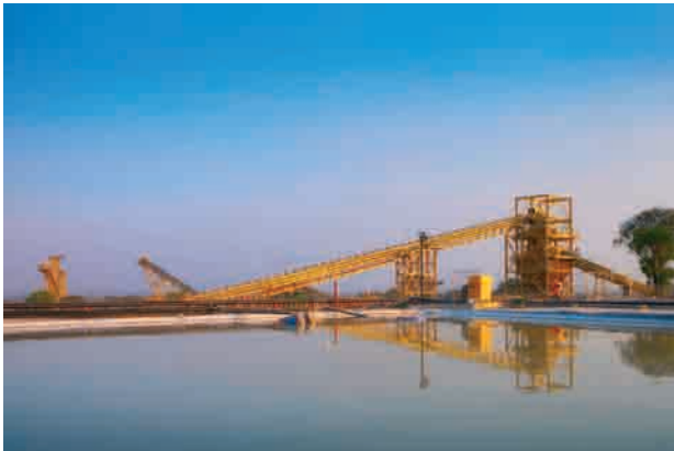
Return water dam with conveyor transfer tower, Lubambe Copper Mine
