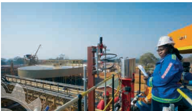
Construction of concentrator plant, Lubambe Copper Mine
