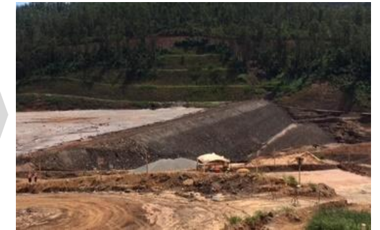
Rebuilt Santarem Dam, March 2016
