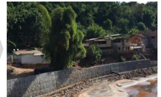
River stabilisation at Barra Longa, May 2016
