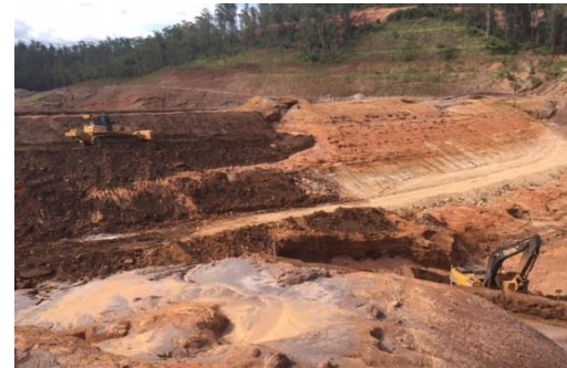
Santarem Dam, November 2015
