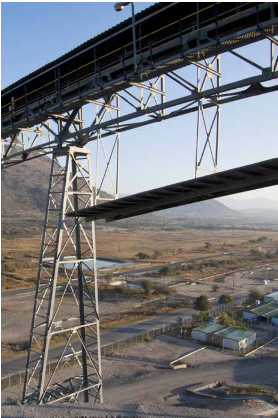
Overland conveyor belt, Two Rivers.
