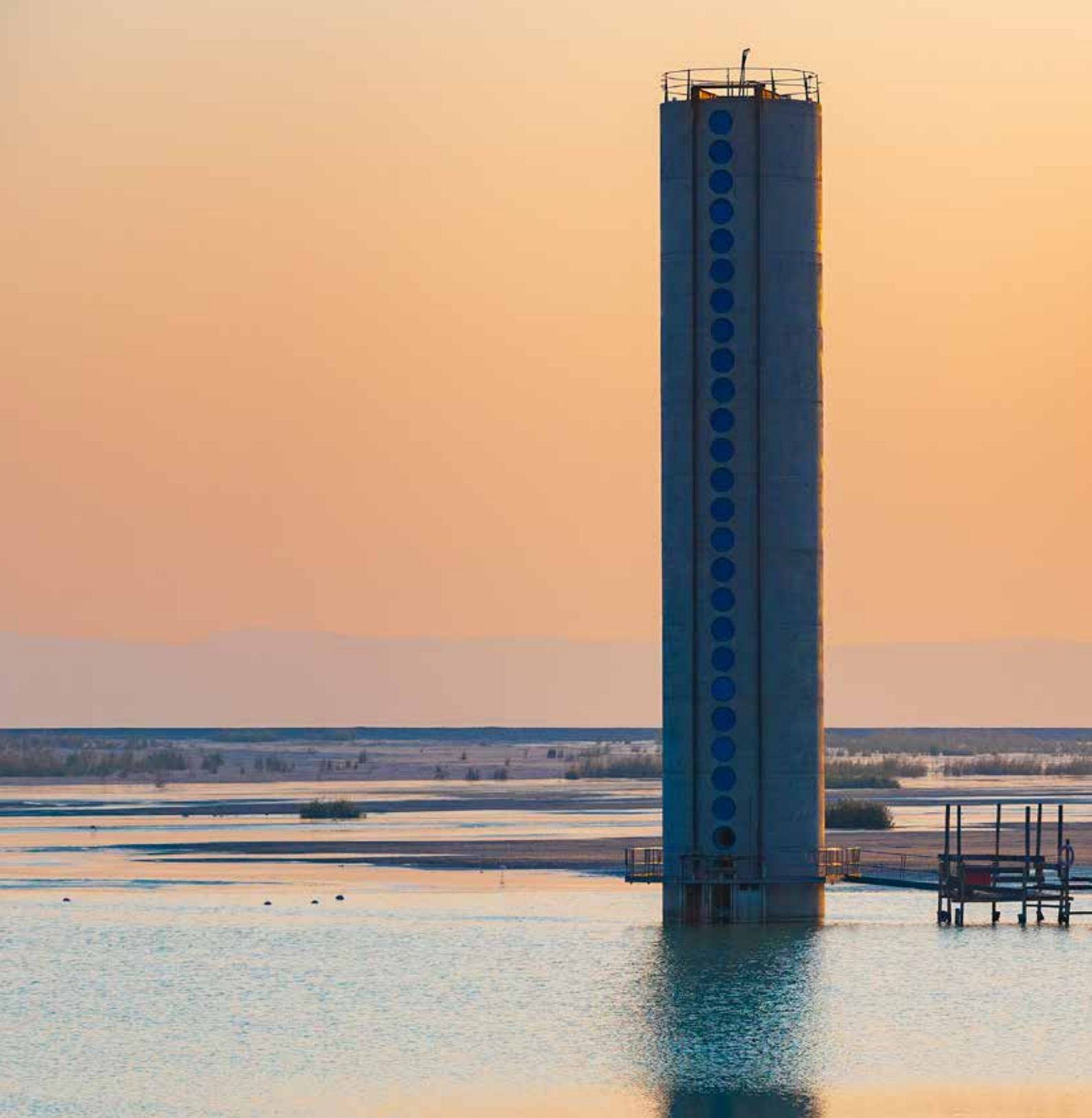
Penstock tower at No 4 tailings storage facility at Impala Rustenburg
