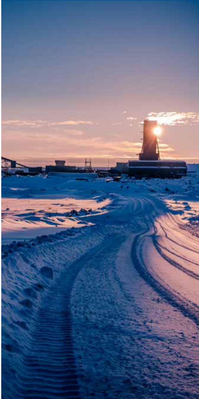
Headgear and surface infrastructure at Impala Canada
