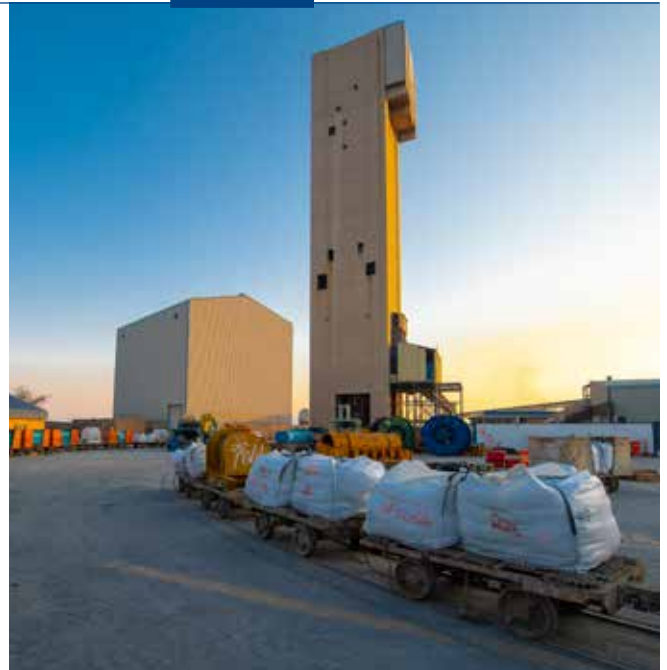
No 16 Shaft headgear at Impala Rustenburg
