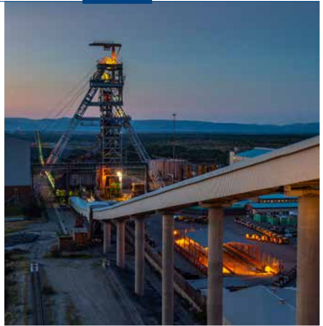
Ore conveyor and headgear at No 14 Shaft, Impala Rustenburg
