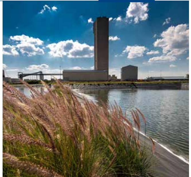
Headgear at number 16 Shaft, Impala Rustenburg
