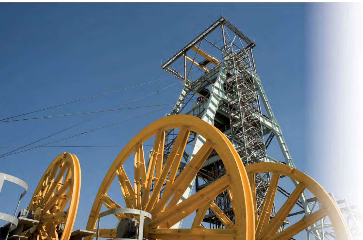
Looking up at 20 Shaft, Rustenburg.
