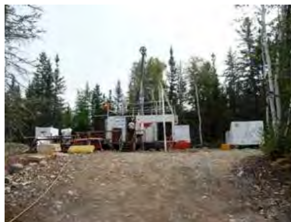
Surface drilling at Milnet/Parkin (Canada)
