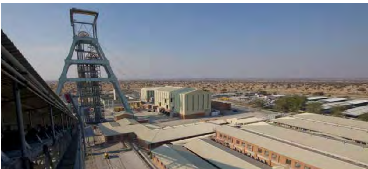
No 20 Shaft, Impala
