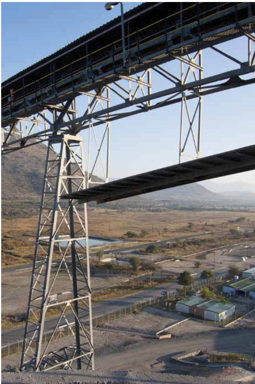
Overland conveyor belt, Two Rivers.
