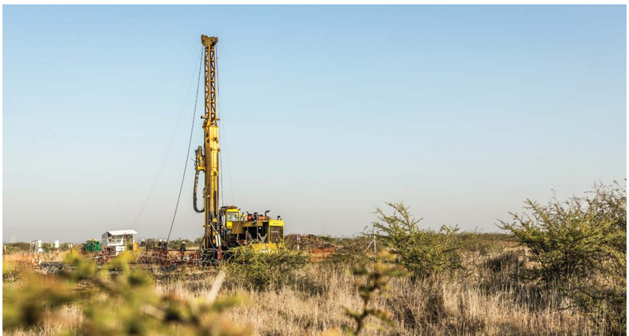
Surface drilling near 16 Shaft, Impala
