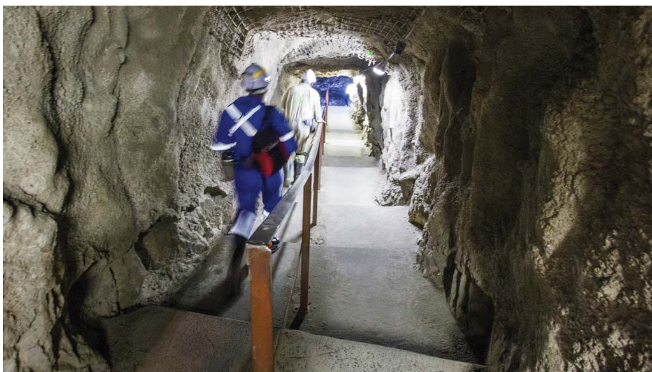
Underground travelling way excavation
