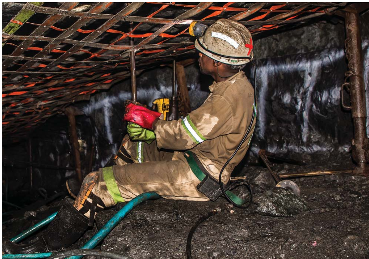
Support installation in a UG2 stope, 12 Shaft, Impala
