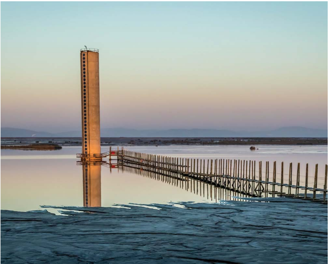
Impala tailings facility
