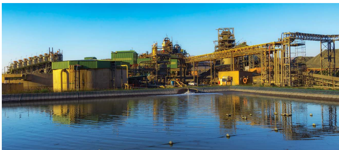
Concentrator Plant – Two Rivers Platinum Mine
