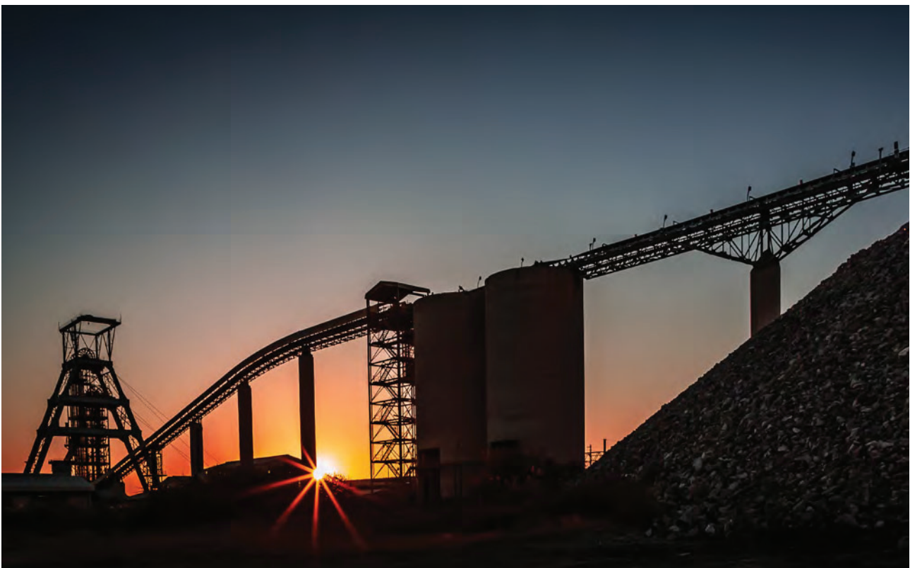
Impala Rustenburg #20 Shaft reef silos and waste dump
