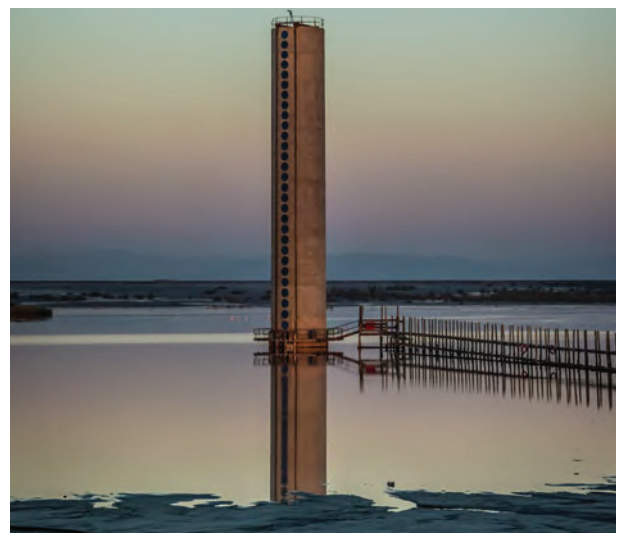
Penstock tower on Tailings storage facility – Impala Rustenburg Photo credit: Jacques McCarthy
