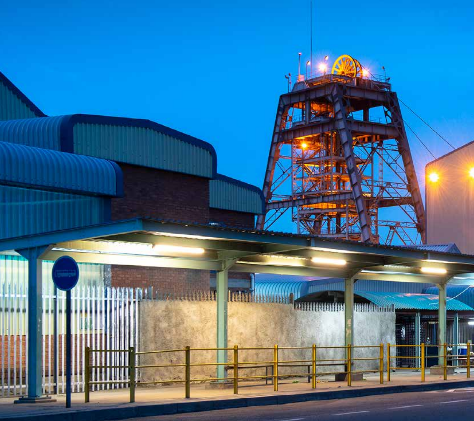
Impala Rustenburg 14 Shaft by night.
