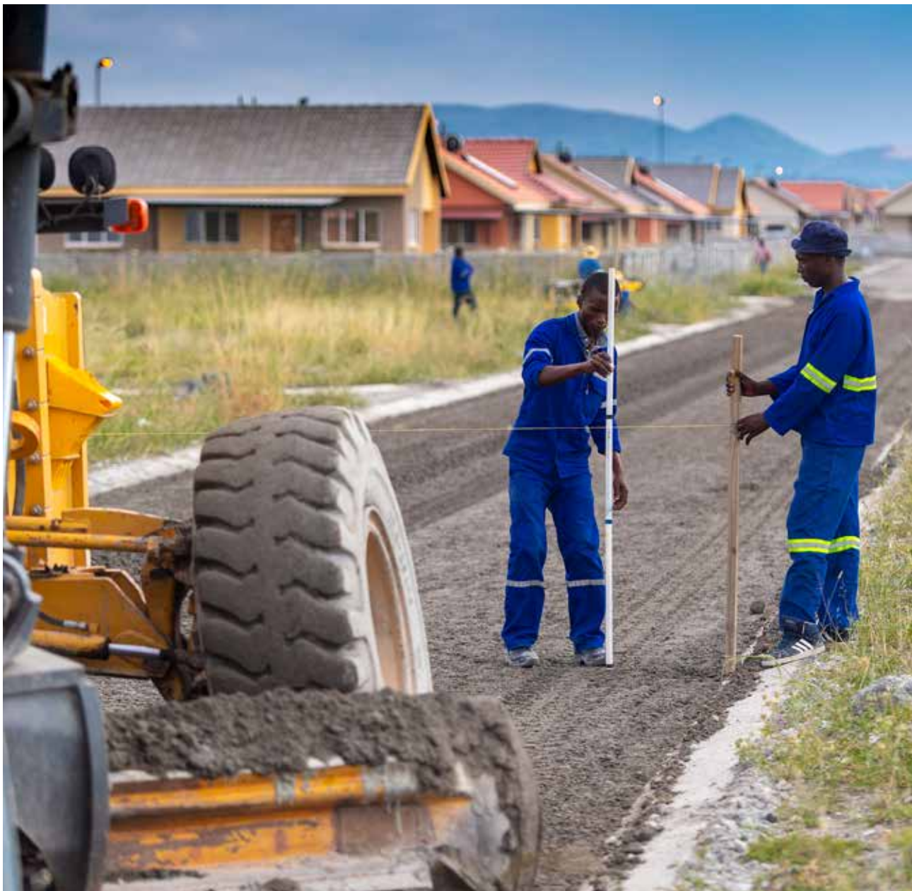
Road construction at Impala Rustenburg's Platinum Village housing development
