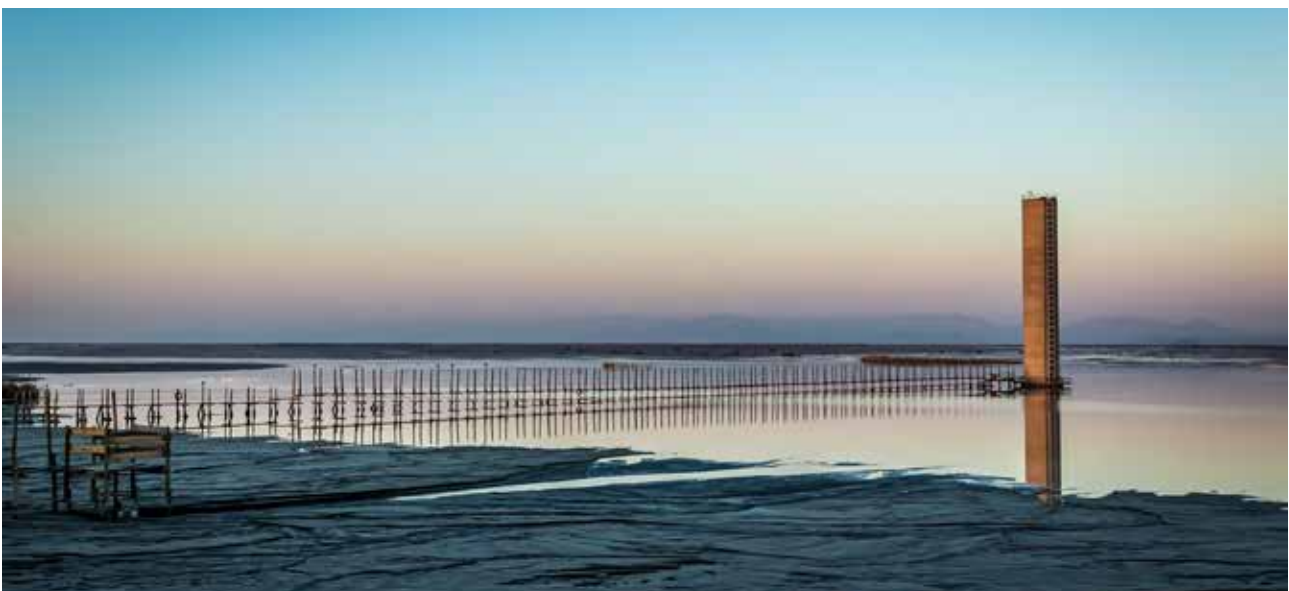
Penstock tower on a tailings storage facility – Impala Rustenburg
