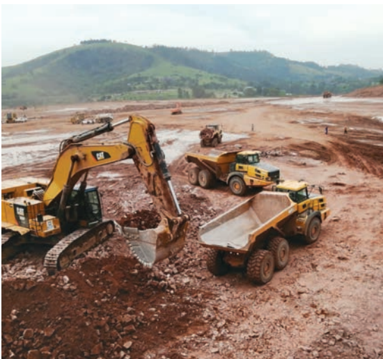
The PEP and Ackermans DC location has the most prominent position on the N3 corridor between Johannesburg and Durban, and is the biggest platform created in South Africa.
