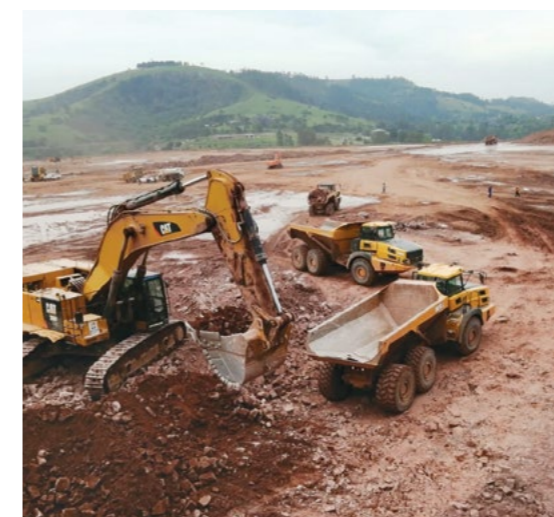
The PEP and Ackermans DC location has the most prominent position on the N3 corridor between Johannesburg and Durban, and is the biggest platform created in South Africa.
