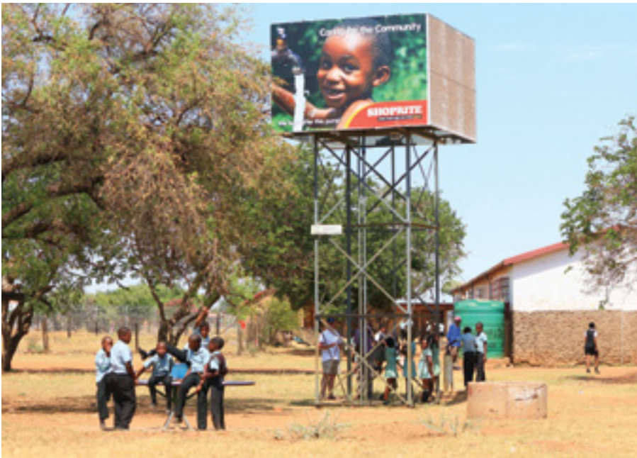
Using advertising space on billboards to fund the PlayPump initiative, in partnership with Roundabout Water Solutions. The initiative has helped 300 000 people at 34 South African rural sites easily access clean water. Water is pumped into a reservoir whenever children play on the merry-go-round.
