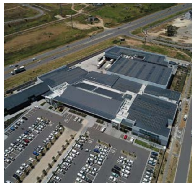
We have increased the installed capacity of our solar PV systems by 350% across 32 sites. This has increased renewable energy generated through rooftop PV systems to 10 993 MWh (2020: 3 298 MWh).
