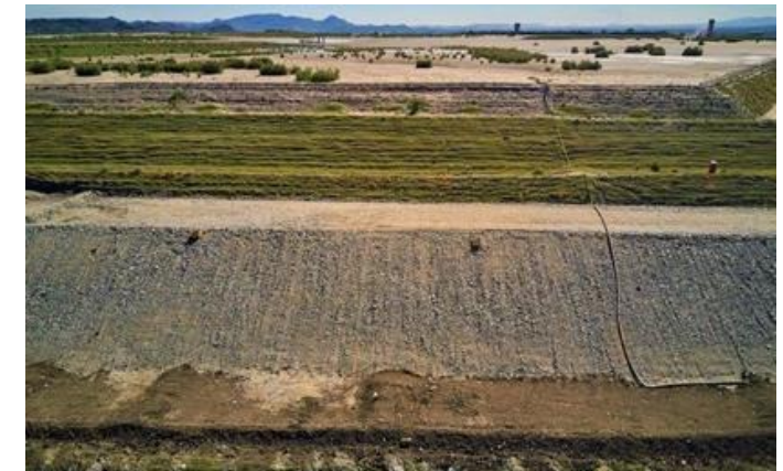
Example of buttressing at SA PGM – Marikana TSF
